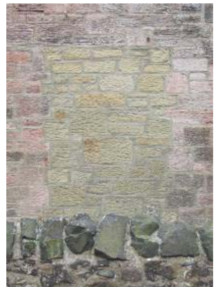
Good work could be better. Left: Good pointing method but a poor mix with insufficient lime. Right: Good match in terms of bonding and stone size, but yellow sandstone is the wrong colour for this area.
